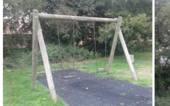
Finding: The timber has a number of air cracks apparent, the splits will have penetrated the preservative applied to the timber and allow water ingress to the unprotected areas
