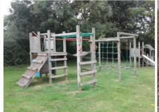
There is some strimmer damage apparent on Action: the posts, this can penetrate the preservative applied to the timber and accelerate the Finding: rotting process
