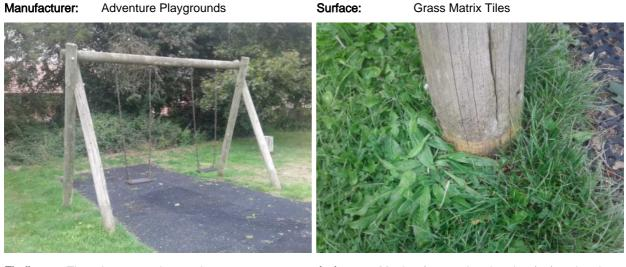
**Finding:** There is some strimmer damage apparent on **Action:** the posts, this can penetrate the preservative applied to the timber and accelerate the rotting process
